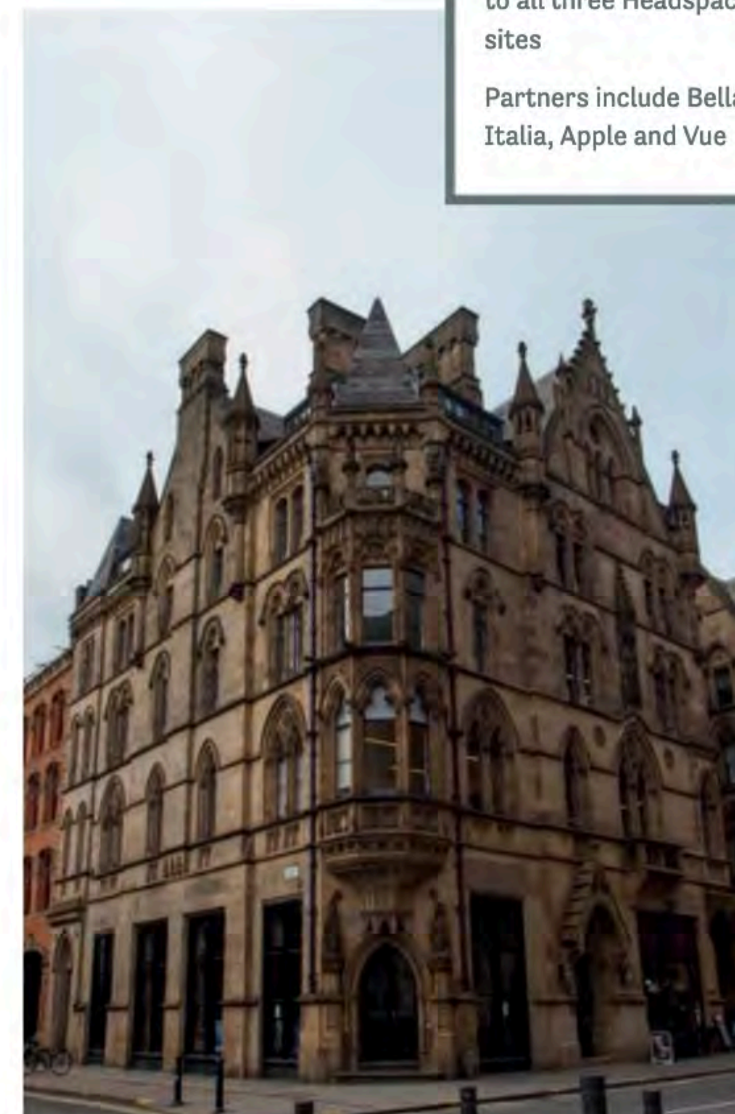
The building is part of the The Albert Estate, a community of dynamic businesses based around Manchester's Albert Square
